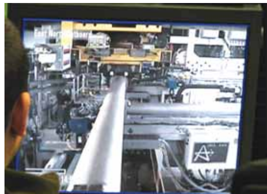
A Retubing Tool Carrier operator remotely transports a loaded transfer can from the receive pallet at the east face to the volume reduction system equipment on the vault floor.
