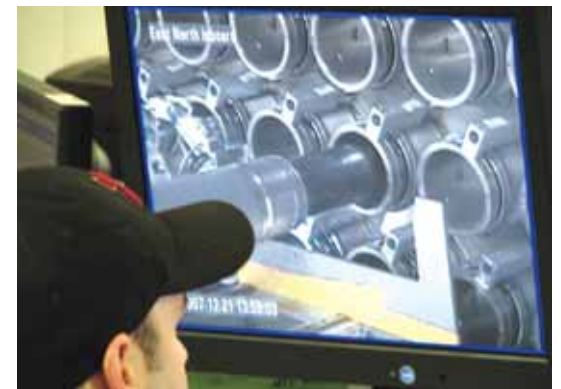
Retube Control Centre Operator Jeff Young observes a close-up of the transfer can inserted into the lattice tube guide sleeve in advance of receiving the pressure tube.
